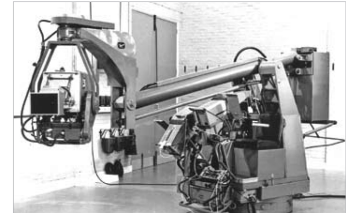
▲ The Peregrine with remote head carrying a full-size 4 1/2" Image Orthicon camera
